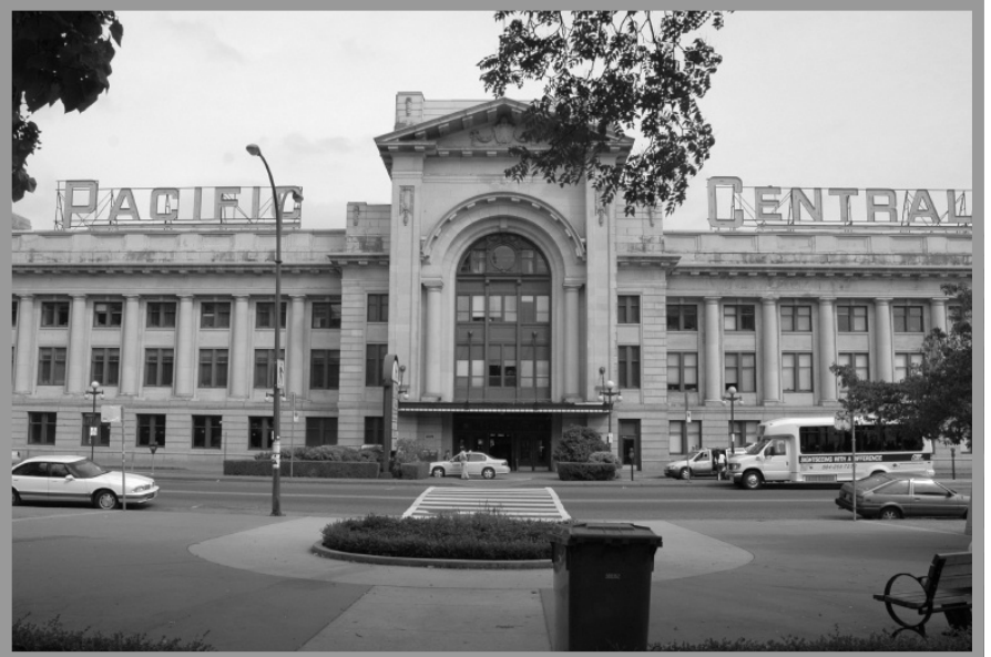
VIA uses the old Pacific Central Terminal in Vancouver, BC. The building has been maintained in excellent condition. It serves the local light rail system as well as Amtrak, so it is a busy place, a nice sight in these days of empty train
